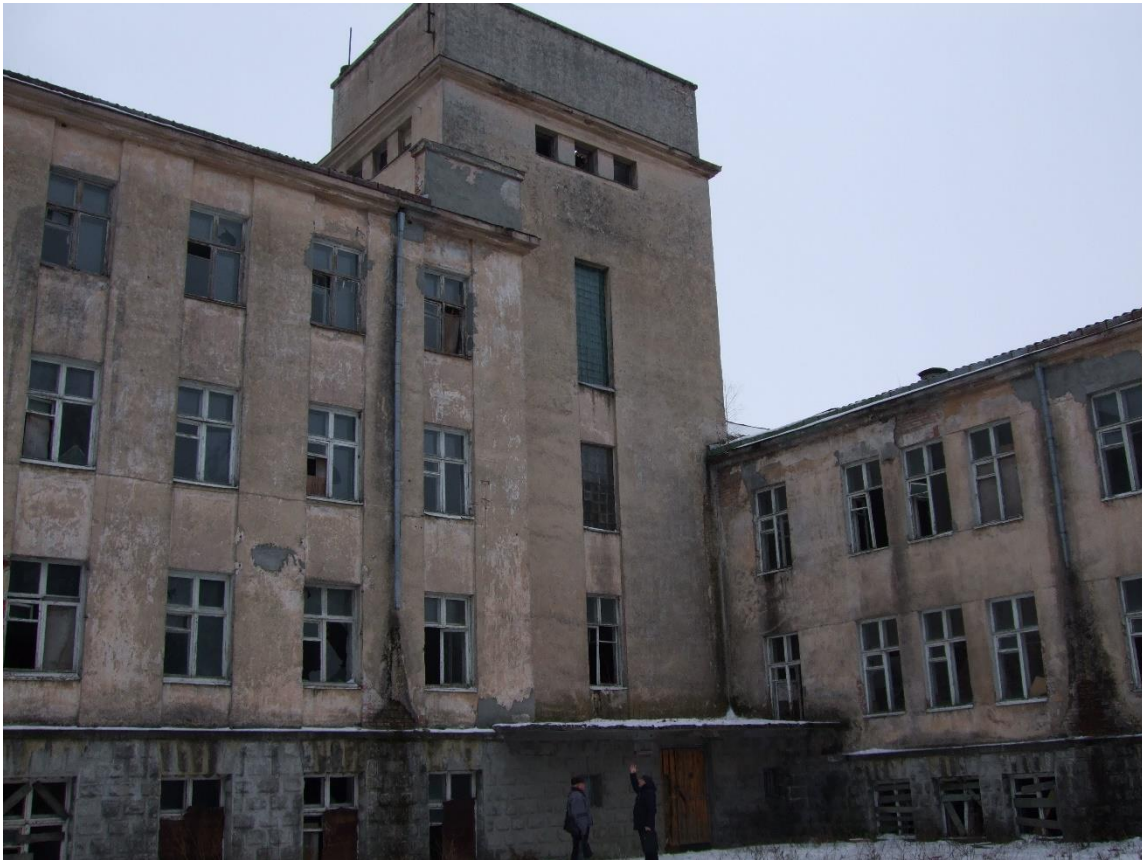
Figure 1. Exterior of the building (Chortkiv, Ternopil Region)
