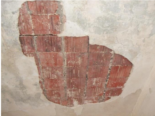
Figure 2. Area “1” Bottom view of hollow block floor on the ground floor
