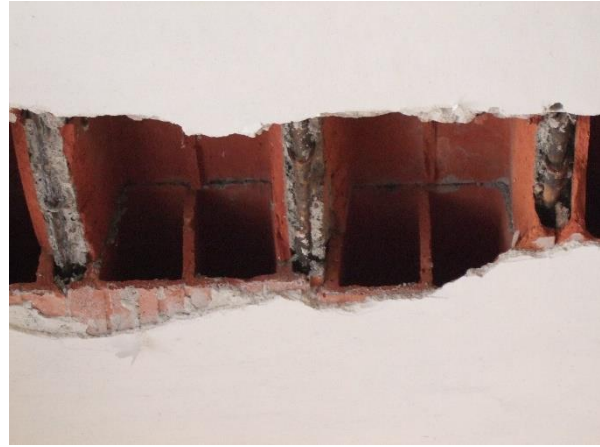
Figure 3. Area “1” Dismantling of bottom surface of hollow block floor on the ground floor
